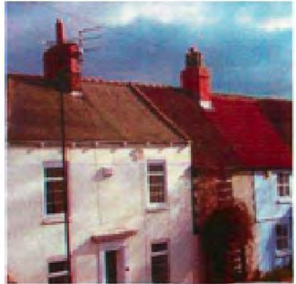
Differing roof materials that can work well together
