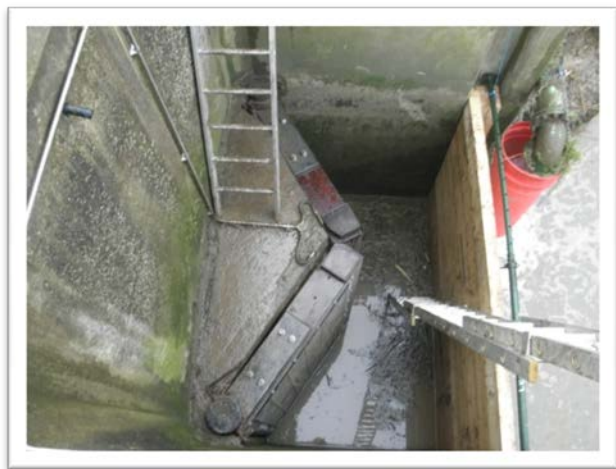
New tidal doors installed
